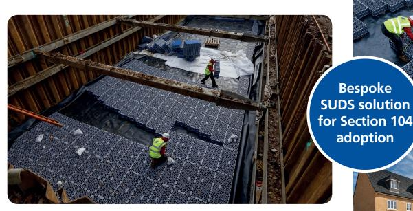
site, with a combined capacity to store up to 558m³ of stormwater.
